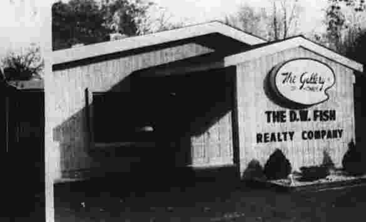
The before and after shots. What was once Fred's Fruitland (nee Burger Chef) at 235 Main St. is now the D.W. Fish Realty Co. Gallery of Homes. It was a major chore to convert the food stand into an office.
